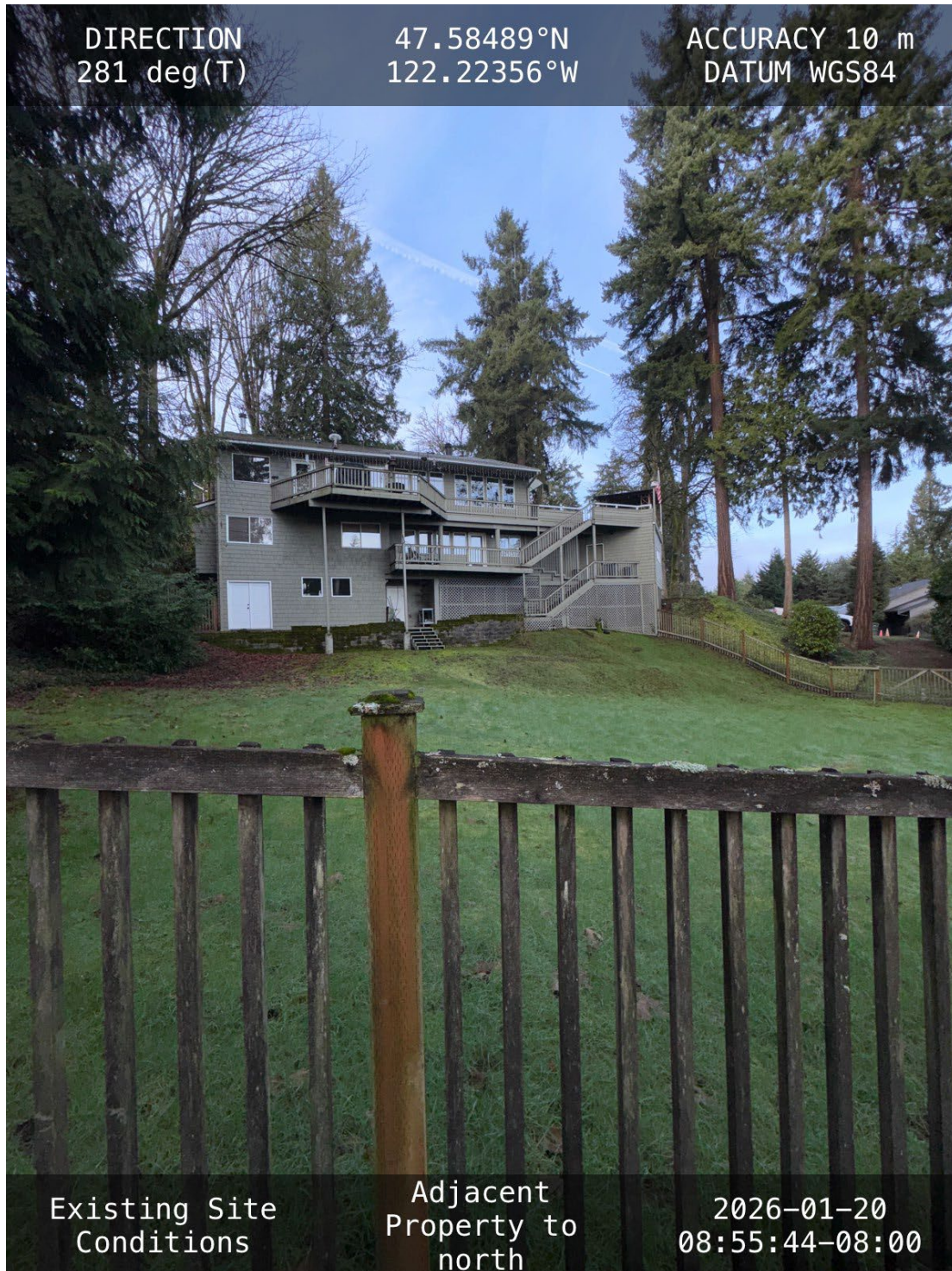
Photo 1. Photo of GIS mapped location of off-Site watercourse (Stream 1) located underground (piped) that continues off-Site through a pipe to the northwest, photo taken facing upslope to the west toward off-Site house.
